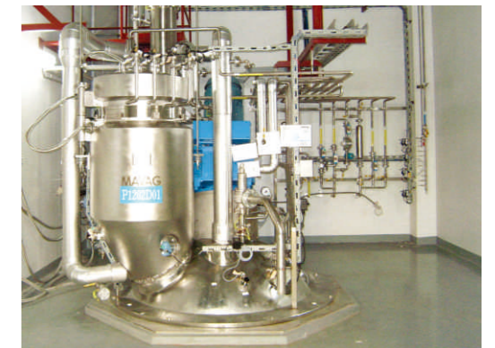
Installed and ready for operation
